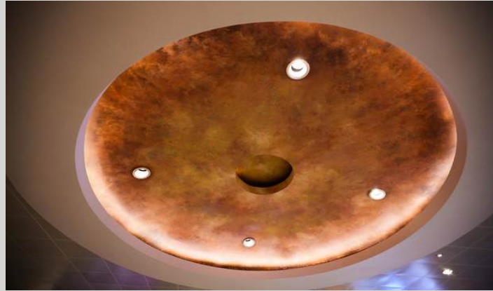
Distressed Copper Ceiling
